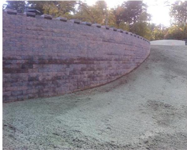
“CURRENT CONDITIONS: Erosion and storm water runoff problems have been eliminated through the installation of retaining walls, a perimeter drain around all the courts and a subsurface drainage system. Additionally, elevation and grading changes have been made to assist with controlling storm water runoff and ponding in sensitive areas.”
