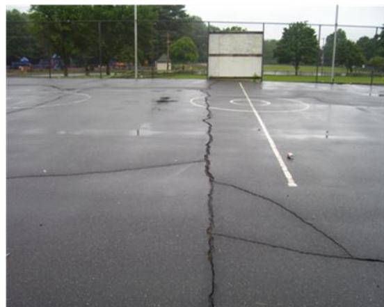
“PREVIOUS CONDITIONS: This was a view looking west showing major cracks within the courts. Each year, due to underlying subsurface conditions, the Courts cracked due to frost heaves and a lack of a proper drainage. The concrete bases, which encapsulate the steel poles that attach to the Tennis
