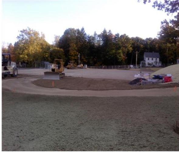
“CURRENT CONDITIONS: This is another view of the new perimeter drain system, the installation of erosion control matting and new grading contours to assist in controlling storm water runoff and eliminating the erosion problems.”
