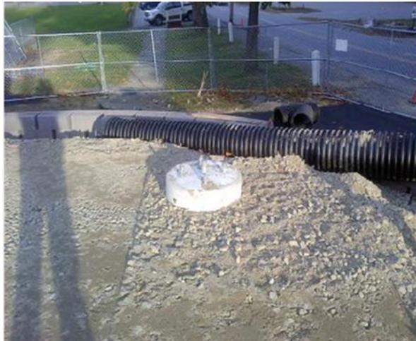
“CURRENT CONDITIONS: These are photos of the installed engineered light pole bases. The tennis courts have 4 bases installed and the basketball courts have 2 installed. All bases were installed with electrical conduits and they are ready for the light poles, fixtures and wiring to be installed, if it is approved tonight.”
