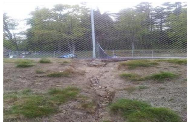
“This is a view looking east and southeast at the previous conditions. Again, the foundation was exposed and there was significant soil erosion. Erosion impacted the surrounding terrain and passive open space areas.”
