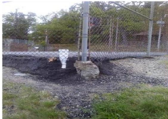
“MORE PREVIOUS CONDITIONS: Here is an example of the deterioration of the old court’s foundation. Without proper drainage, storm water runoff contributed to the continual erosion problems. As you can see, the concrete base of the existing fence pole was exposed and the foundation was crumbling. Storm Water runoff and erosion impacted the areas below the courts near the Concession Stand.”
