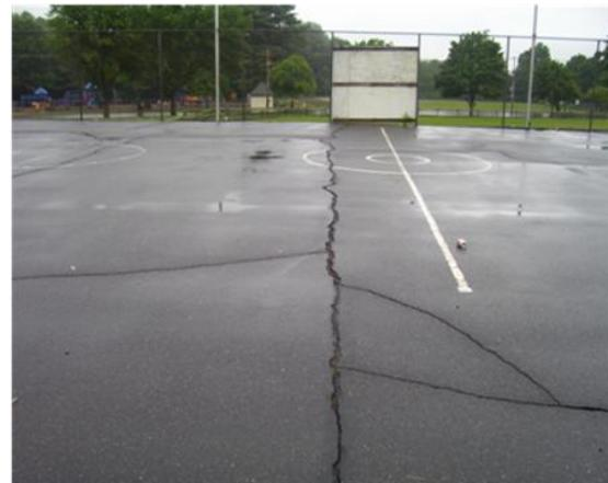
“PREVIOUS CONDITIONS: This was a view looking west showing major cracks within the courts. Each year, due to underlying subsurface conditions, the Courts cracked due to frost heaves and a lack of a proper drainage. The concrete bases, which encapsulate the steel poles that attach to the Tennis
